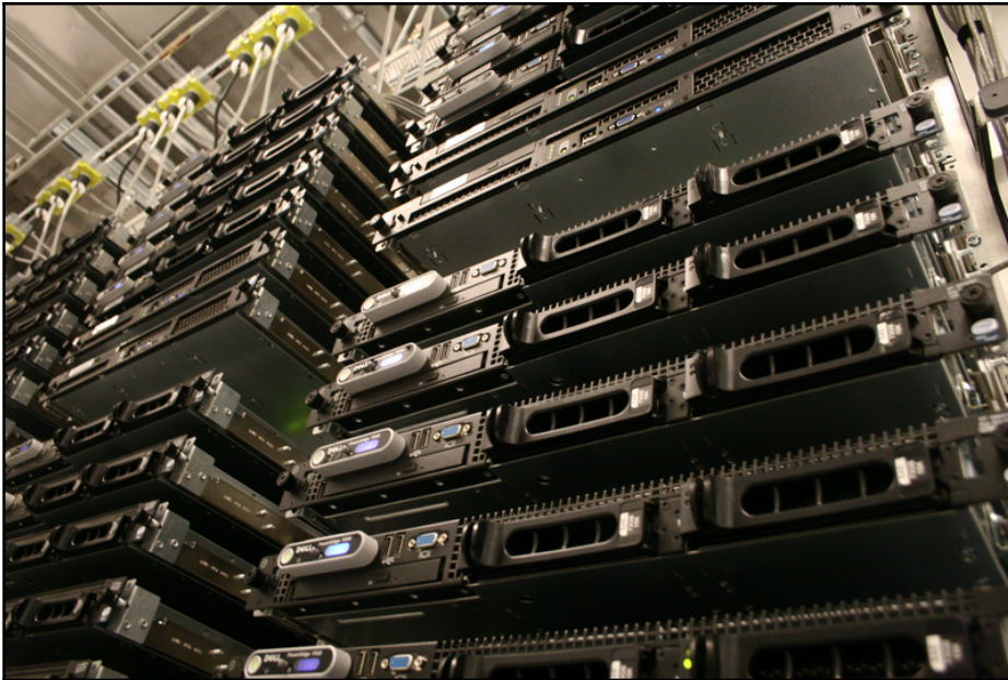
1U rack servers installed in a rack system Image courtesy: 2018 FatCow Web Hosting
