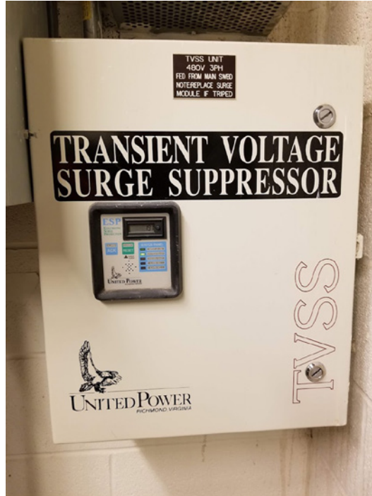
FIGURE 22.16 An industrial service entrance surge protection unit
